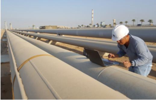
Based on inspection data, pipeline integrity engineers can provide a complete integrity assessment of the pipeline. Individual corrosion features are assessed on their severity and potential risk.
